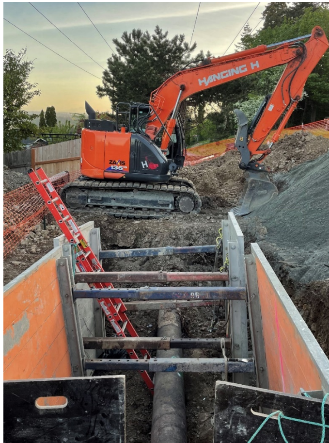
Figure 9 – Excavation of the Olympic Pipeline in Somerset, May 2021
