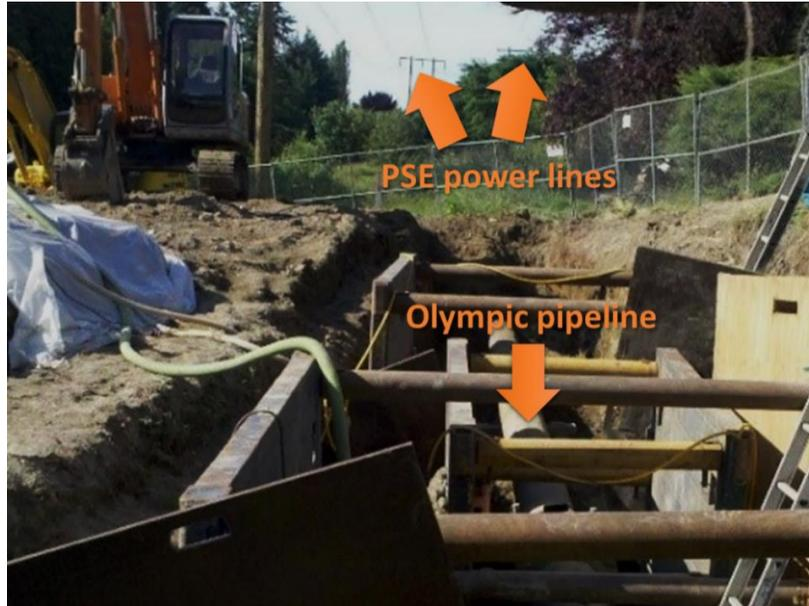
What would happen if a line with double the voltage and higher current fell near the pipeline? We don't know, but it's possible that a powerful electric arc could pierce the pipeline casing in a relatively short time, unleashing a "catastrophe" (in the words of the Bellevue Fire Department) that could not be extinguished by local firefighters using normal equipment.
